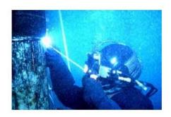
In wet welding MMA (manual metal arc welding) is used.
